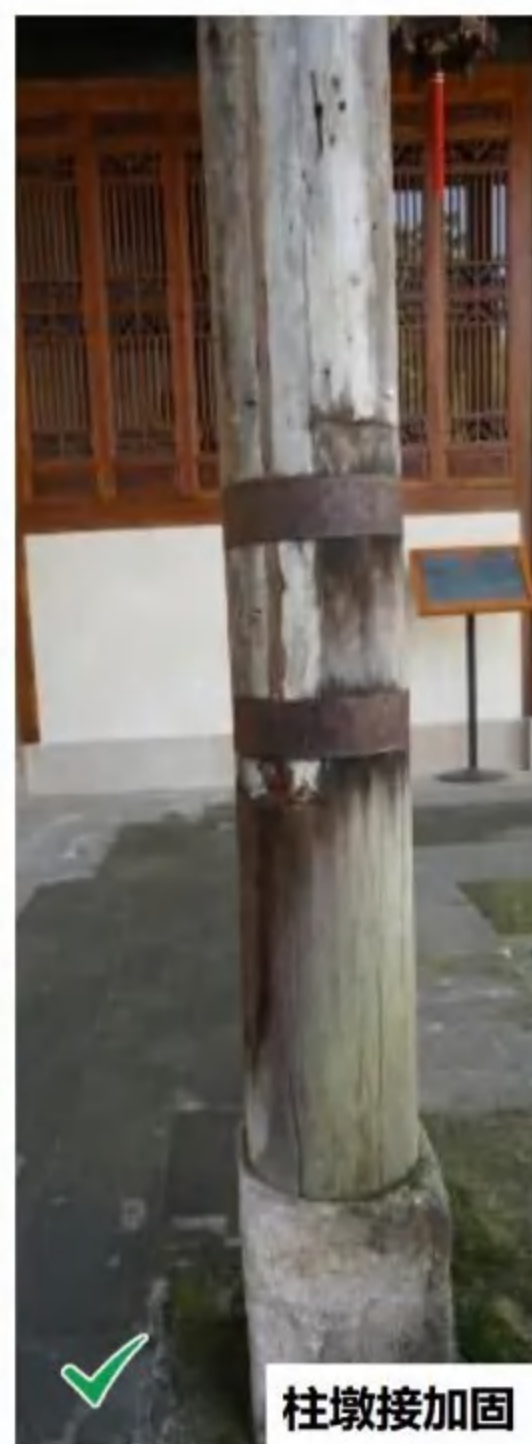
柱根腐朽
